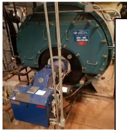
Direct Install can be used for energy-saving upgrades to lighting; heating, cooling & ventilation (HVAC); refrigeration; motors; natural gas and variable frequency drives.
