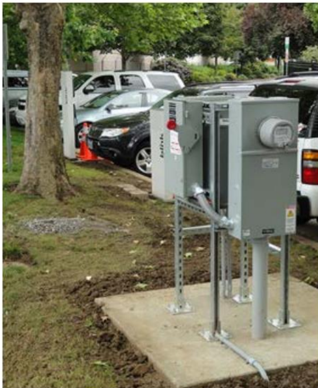
Electrical meter and switch servicing Level 2 EVSE. Photo from Don Karner.
