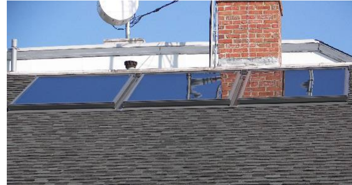
Manchester, NJ solar thermal installation
