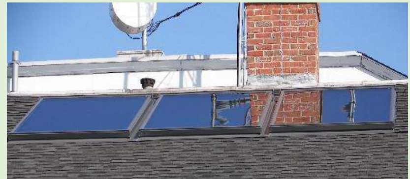
Manchester, NJ solar thermal installation
