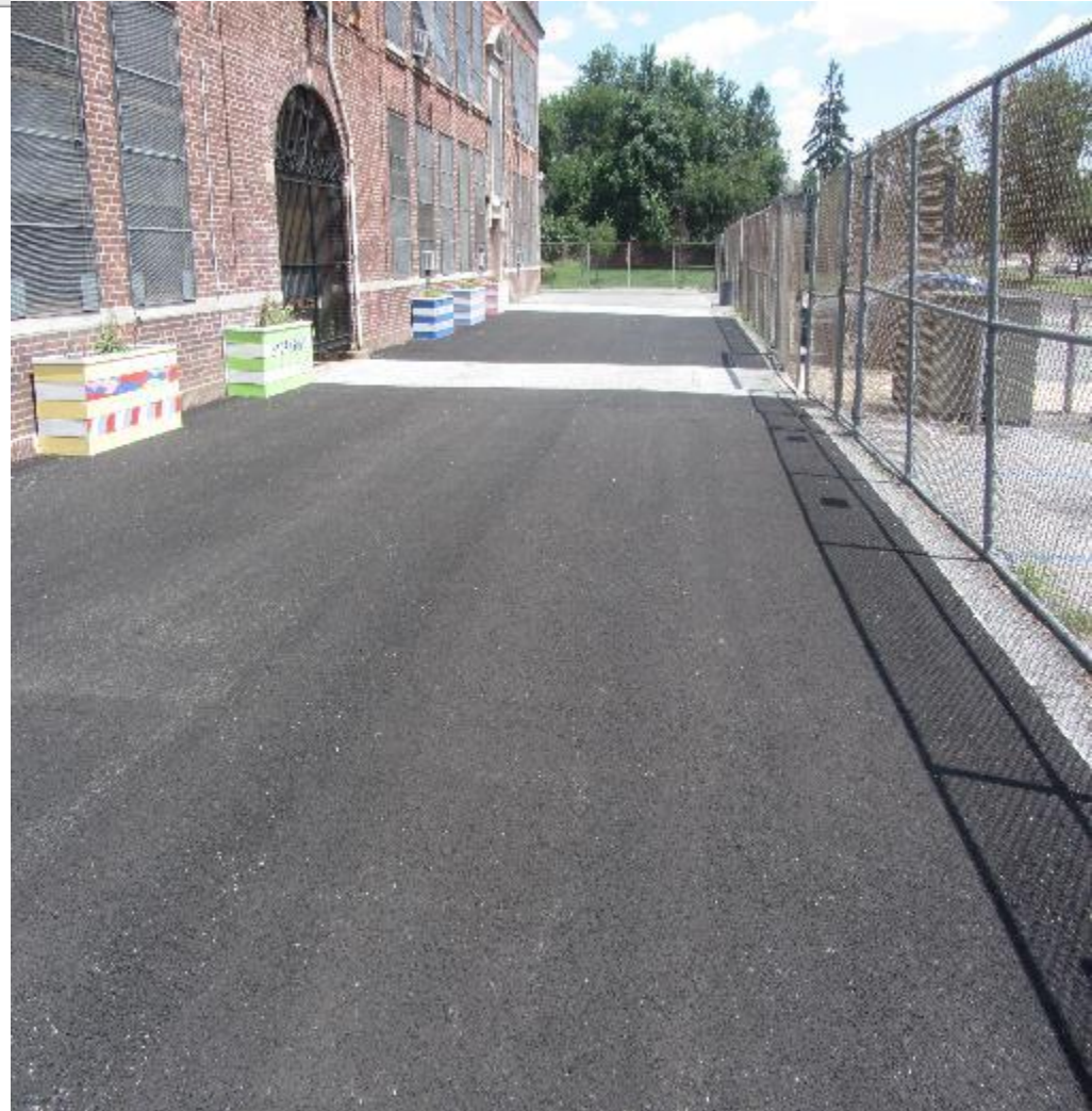
Porous Pavement (Asphalt) at Yorkship School in Camden, NJ Storage System
