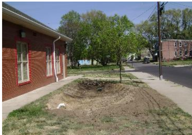
Rain garden installation at Ferry Avenue Library in Camden, NJ Vegetative System
