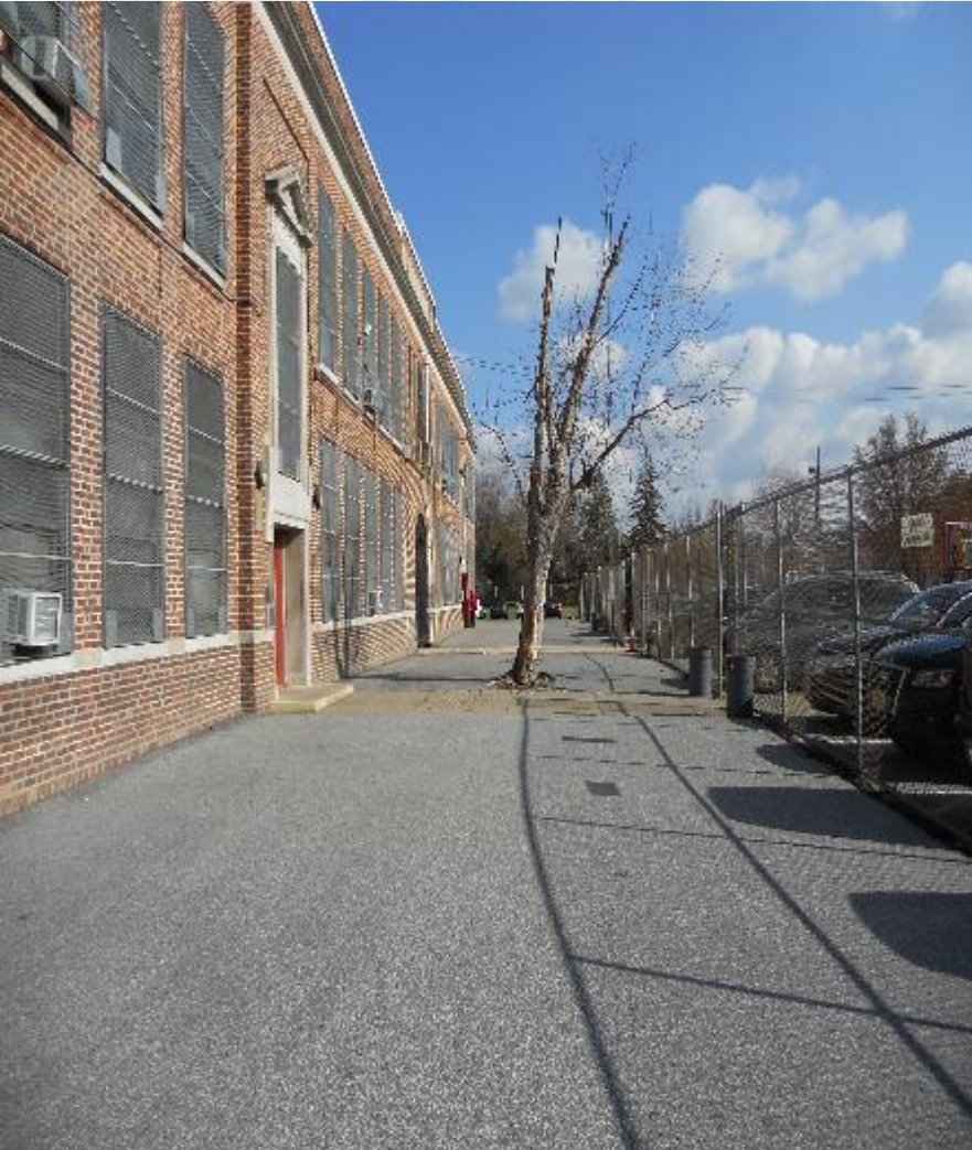
Porous Pavement (Asphalt) at Yorkship School in Camden, NJ Storage System
