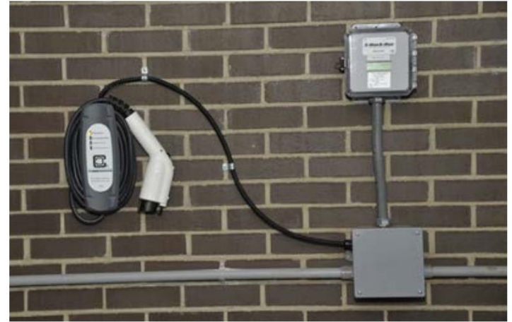
Photo 4. Wall mounted EVSE installed by the New York Power Authority for employee charging. Photo from NY Power Authority, NREL 26468.
