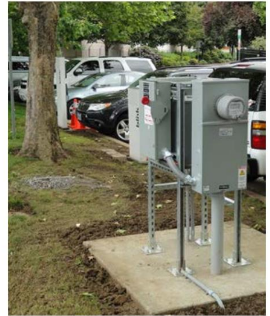
Electrical meter and switch servicing Level 2 EVSE. Photo from Don Karner. https://afdc.energy.gov/files/u/publication/evse_cost_report_2015.pdf
