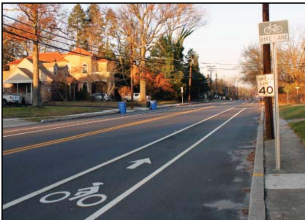
Cherry Hill and Camden County partnered to install bicycle lanes on Kings Highway before either entity had adopted a Complete Streets policy
