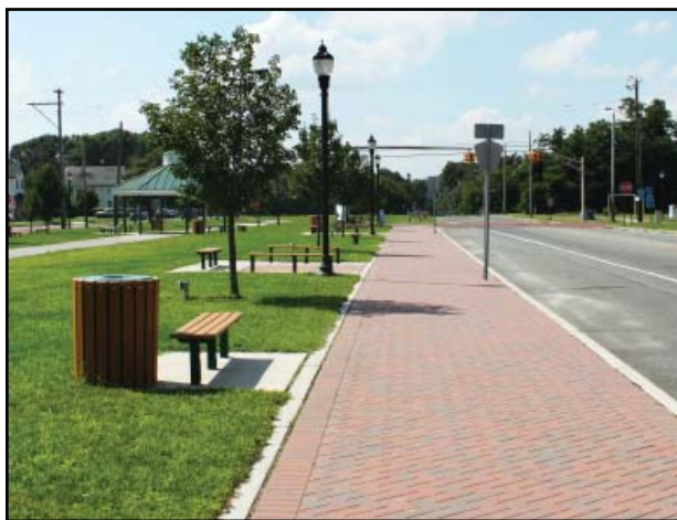
Streetscaping improvements on Dehirsch Avenue
