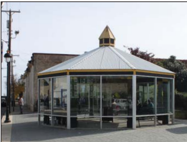
New transit shelter at Pleasantville bus terminal
