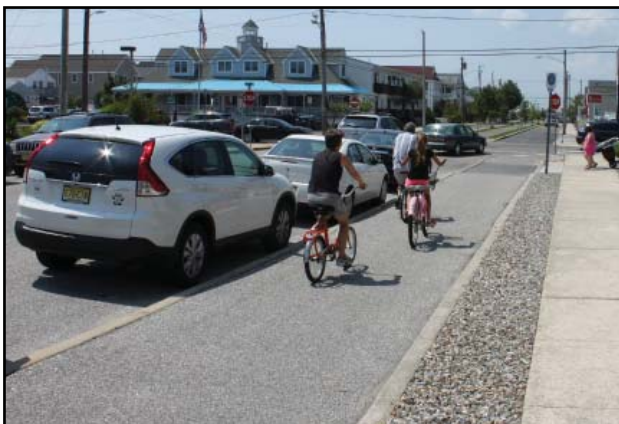
Cycle-track on Haven Avenue, adjacent to parked vehicles, physically separates bicyclists from motorists and pedestrians
