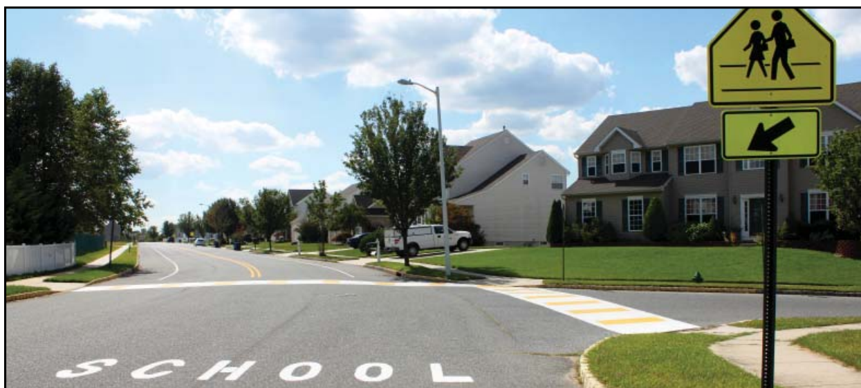
Sidewalks, high-visibility crosswalks, and signage in a residential school zone in Woolwich Township
