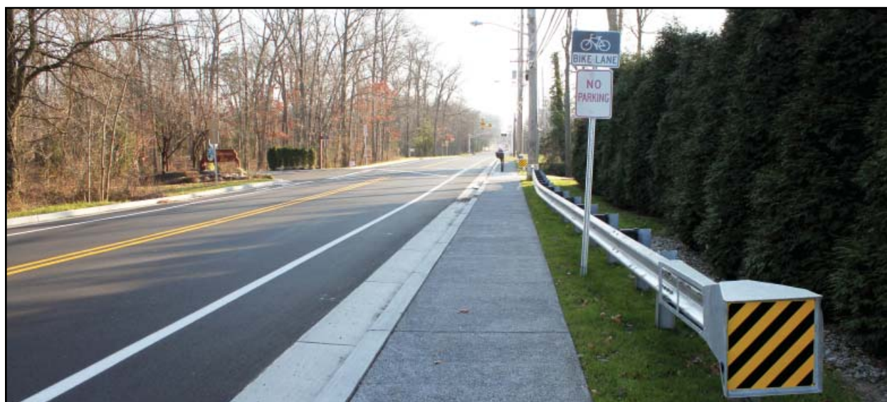
New sidewalk and bicycle lanes on Springdale Road (CR 673)
