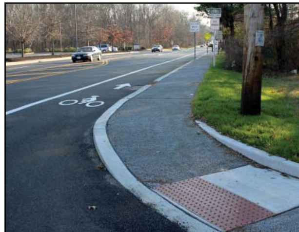
Newly installed sidewalk and bicycle lanes on Springdale Road (CR 673)
