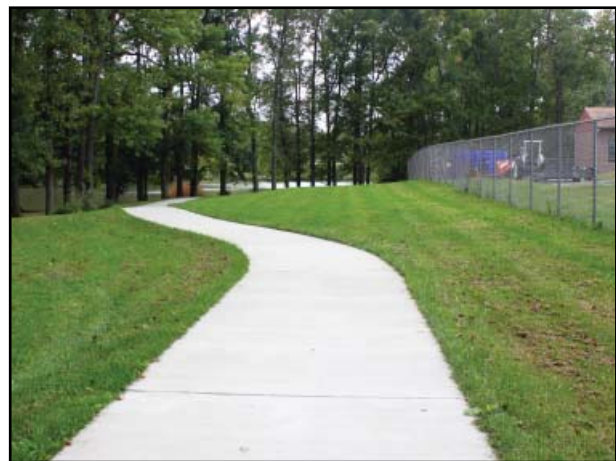
Recently constructed multi-use trail in Stewart Park
