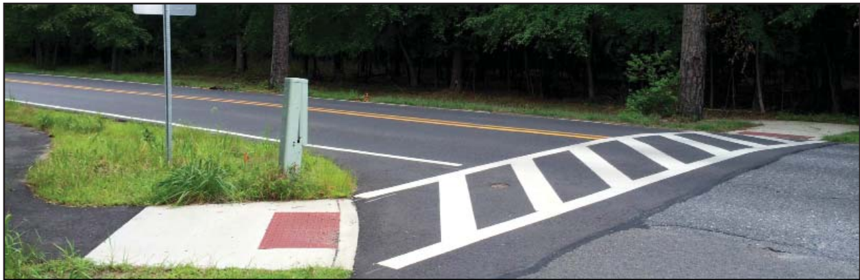
High-visibility zebra crosswalk and ADA-compliant curb ramps on Fairview Road at Woods Drive
