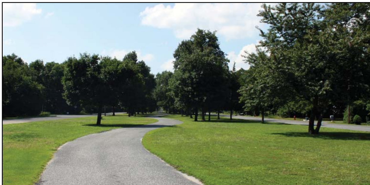
Multi-Use Path on the median of Dehirsch Avenue in Woodbine
