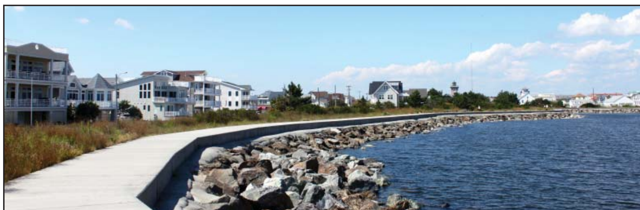
Seawall pedestrian path
