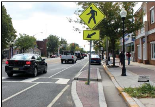
New bicycle lanes and crosswalks on Route 45 (North Broad Street) in Downtown Woodbury
