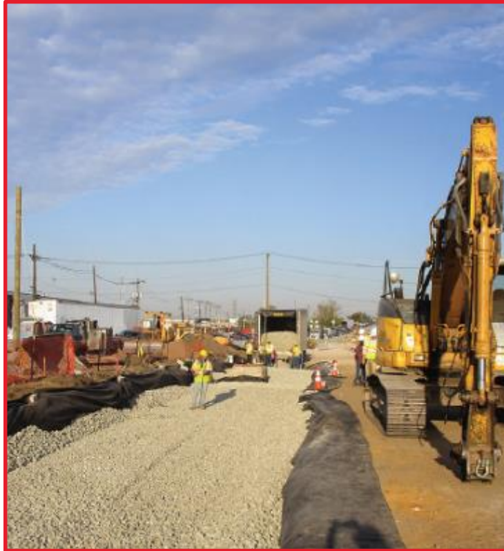
Foam glass aggregate used on the Route 7 Wittpenn Bridge project
