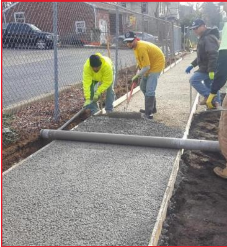
Porous Concrete on Westfield Ave., Camden City
