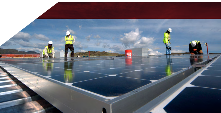
NREL. 2012. Solar Installation. Photo by Dennis Schroeder. 21512.
