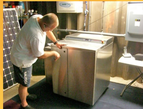
Electrolyzer and Hydrogen fuel cell
