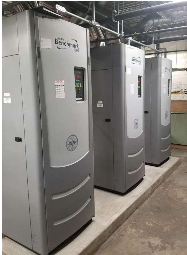
Neptune High-efficiency boilers
