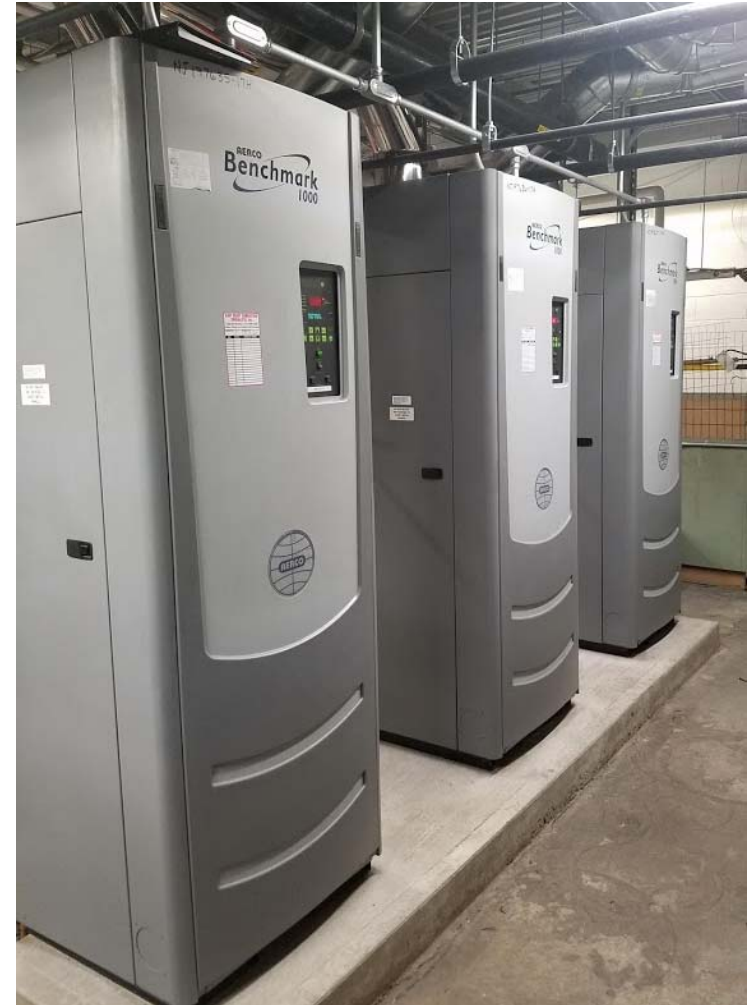
Neptune High-efficiency boilers
