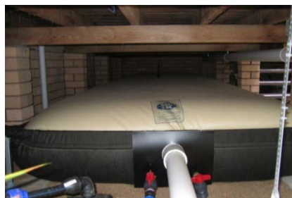
Rain Bladders & Cisterns
