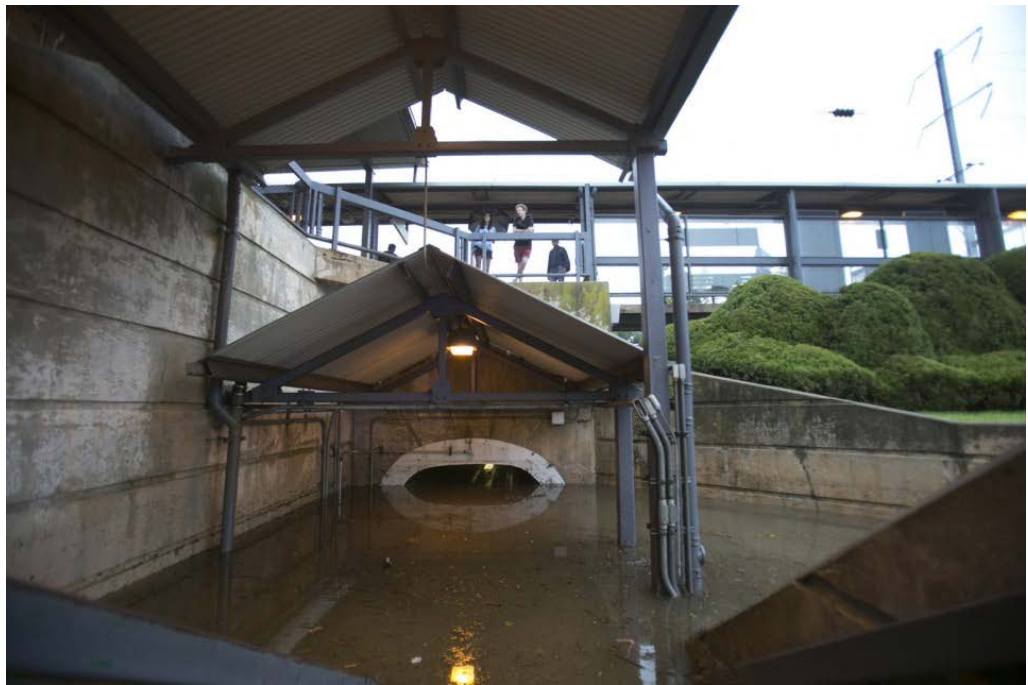
Princeton Junction after 7”+ of rain, July 2016
