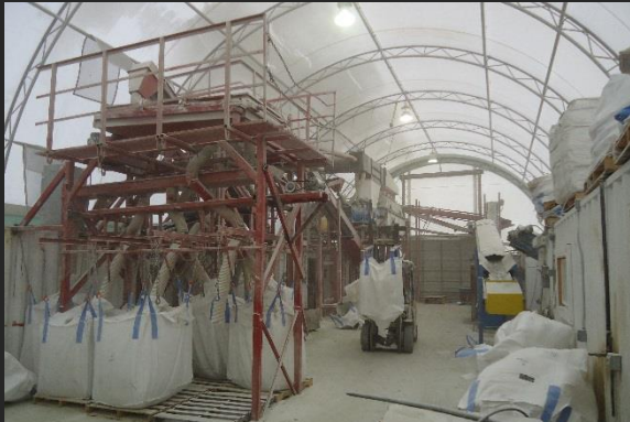
Pilot Plant Richfield Springs NY
