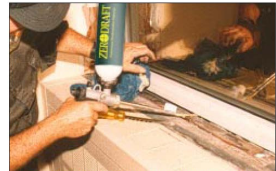
Zerodraft Foam Sealant being applied to seal gap between window frame and rough opening.
